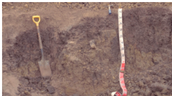
Excavation at site of SW82 and SW83
